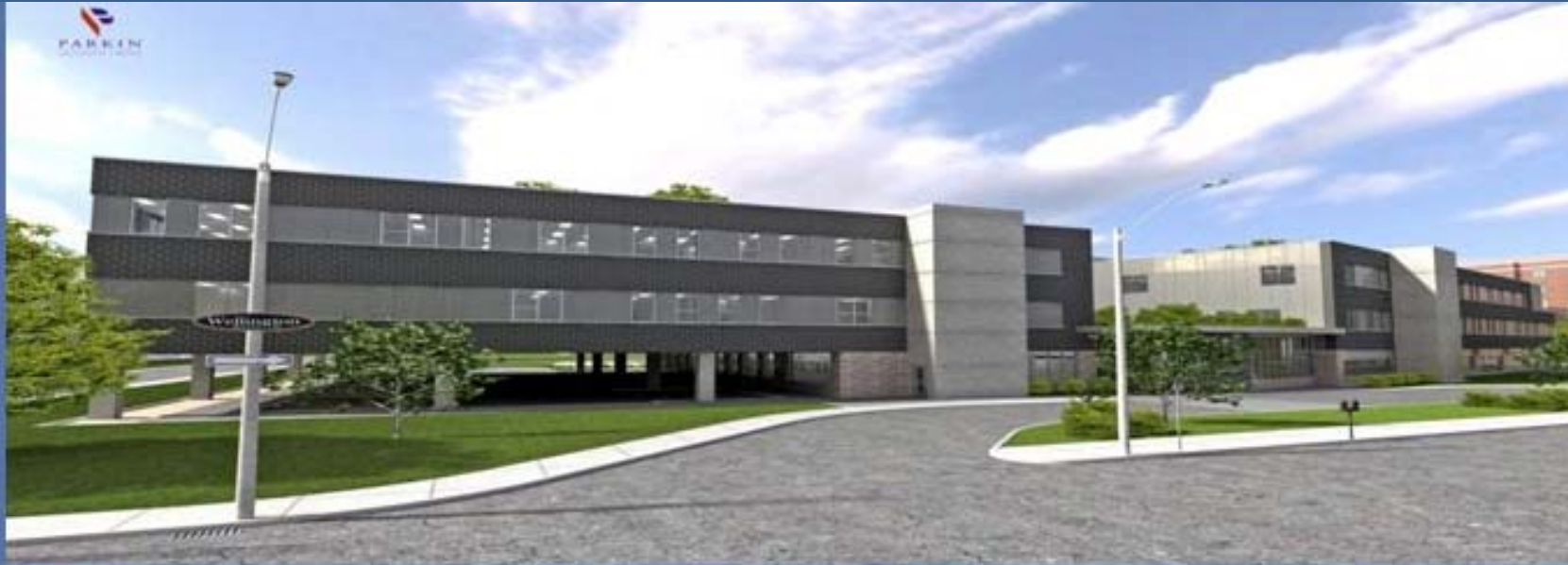
Front Entrance (West Elevation)
