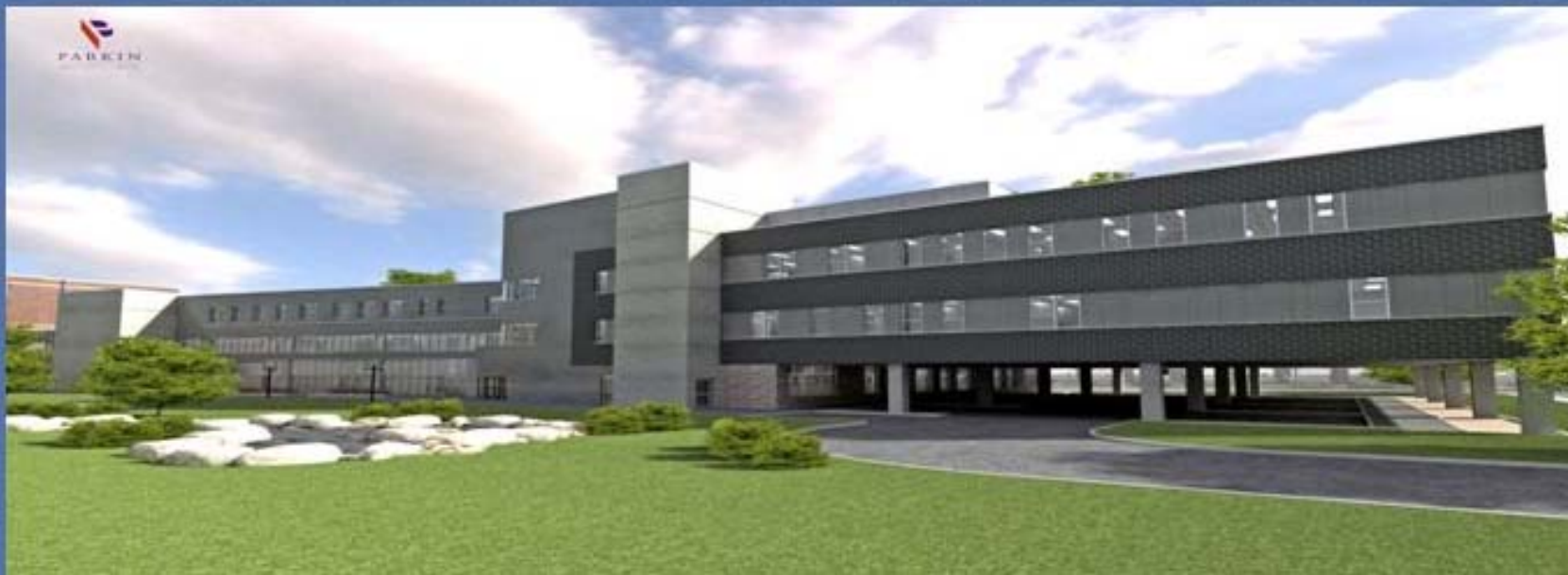
Wheeling Track (East Elevation)
